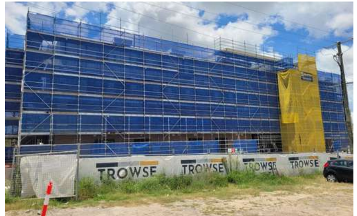
508 Chambers Flat Road Four storey school building almost completed
