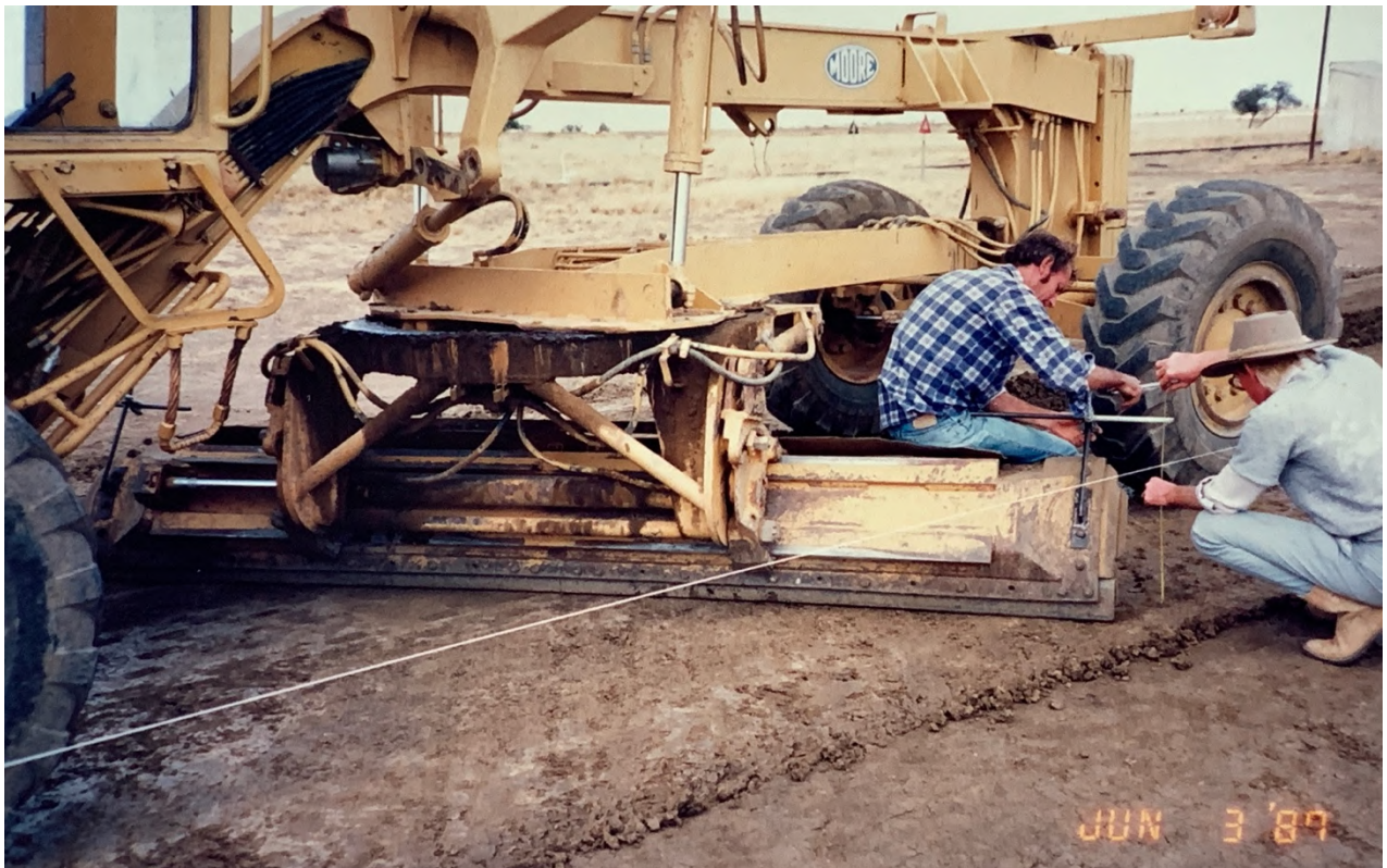
Adjusting the height of the pointer on the grader blade. (Winton Shire)
