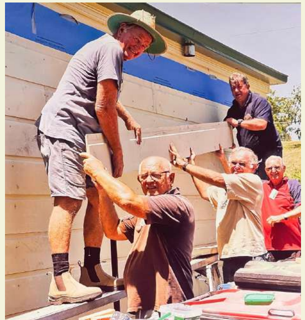
Cladding the external walls
