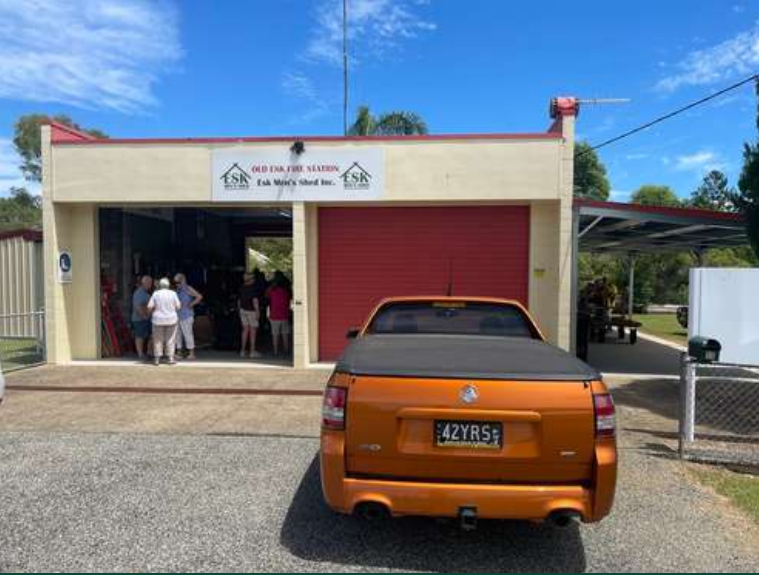
Esk Men's Shed - the old Fire Station building
